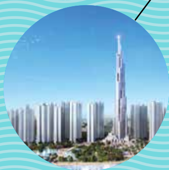
Heat pumps Vinhomes Central Park Vietnam
