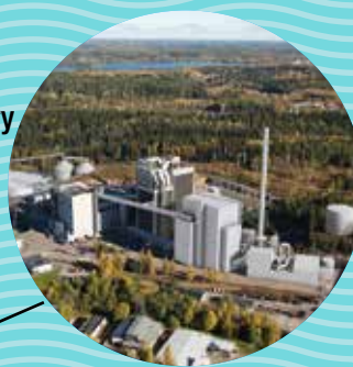
Burners Kymijärvi III, bioenergy heating plant Finland
