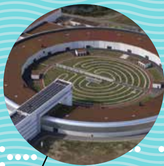
Heat pumps MAX IV, particle accelerator laboratory Sweden
