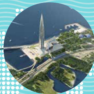
Burners Lakhta Center Russia
