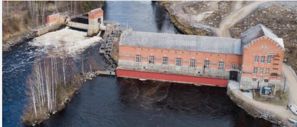
Project: Kuhankoski hydroelectric plant Oilon's customer: Lämpöpalvelu Sami Päijänen Heat pump: RE 96 Total capacity: 96 kW Heat source: power plant cooling pond Number of heat pumps: 1 Location: Laukaa, Finland
