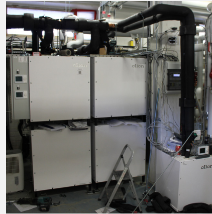
Project: AS Oy Relanderinaukio 4 Oilon's customer: Suomen Kiinteistölämpö Oy Heat pump: RE 96, ECO 21 Total capacity: 213 kW Heat source: boreholes Number of heat pumps: 3 Location: Helsinki, Finland
